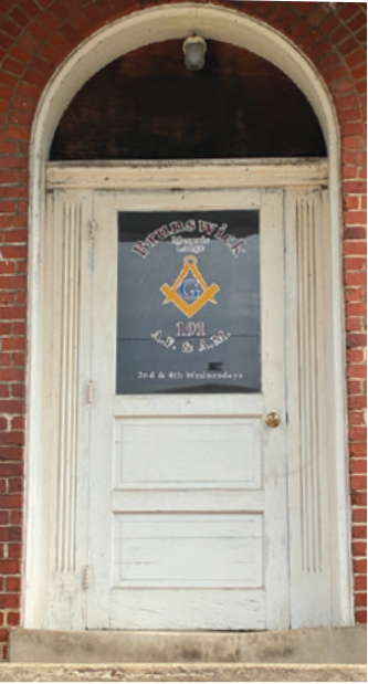
For over 70 years, members of Brunswick Masonic Lodge #191 passed through this door at 321 Brunswick Street.
