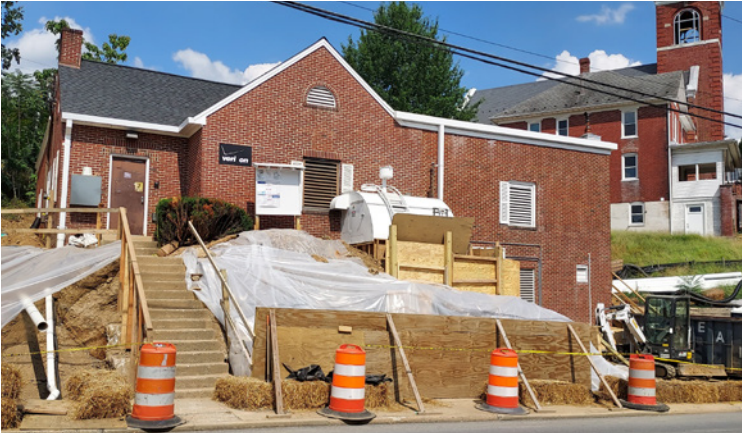
Verizon building undergoing very slow-going improvements.
