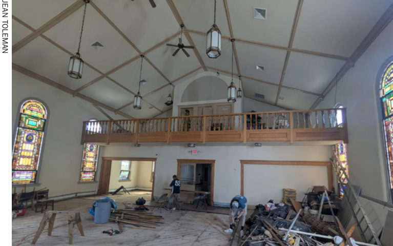
Removal of floor and interior structures in First Baptist Church nearing completion.
