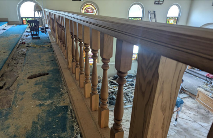
Looking from the balcony down into the church with flooring removed.
