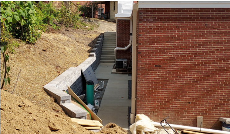
Improvements to the rear of the building.
