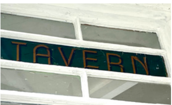
The lettering “Tavern” on a small transom window was hidden by paint for many years, but was revealed and preserved during the rehab.
