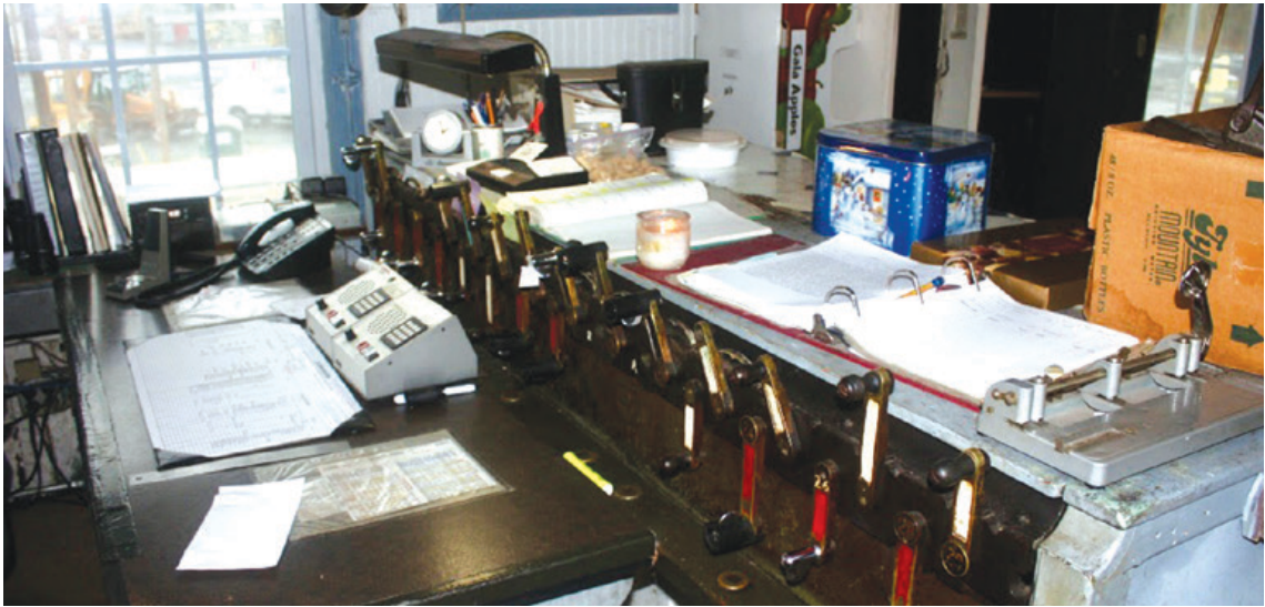
US&S Model 14 pneumatic interlocking machine in the WB Tower.
