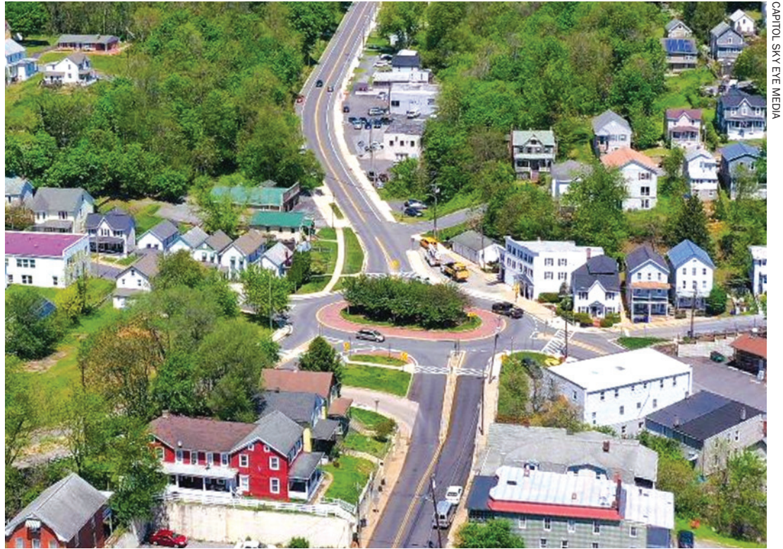
Brunswick's first roundabout where Route 17, Petersville Road, B Street and Maryland Avenue all come together.
