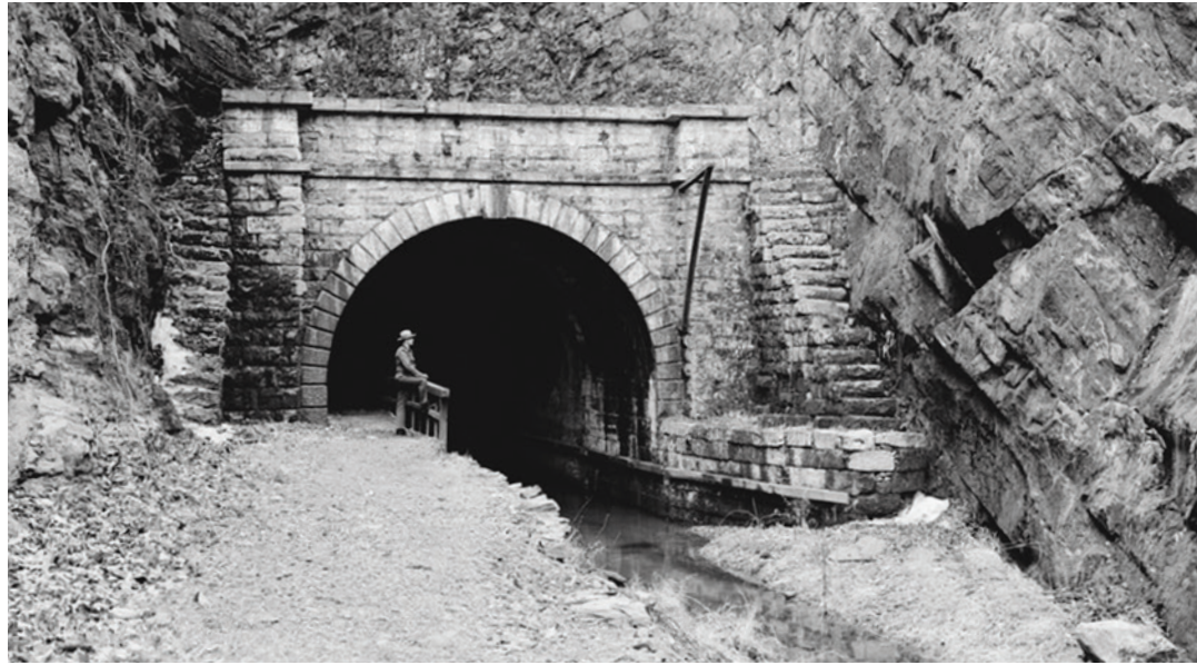
North portal of the Paw Paw Tunnel, with a ranger on the towpath.
