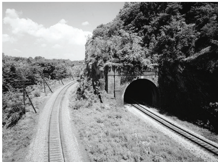
South portal of the Point of Rocks Tunnel.
