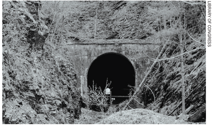
East portal of the Stickpile Tunnel.
