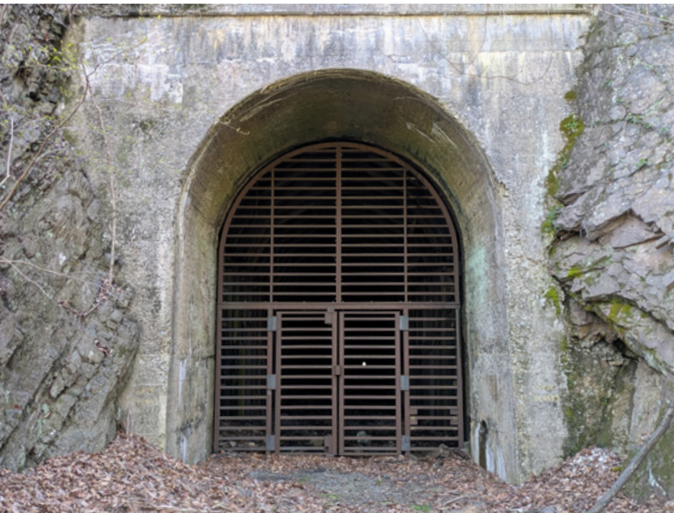
The Indigo Tunnel on the Western Maryland Rail Trail just beyond Sideling Hill.
