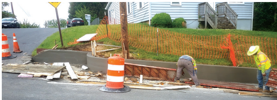
Workers preparing to add new sidewalk to a segment that had none. The retaining wall was also replaced.
