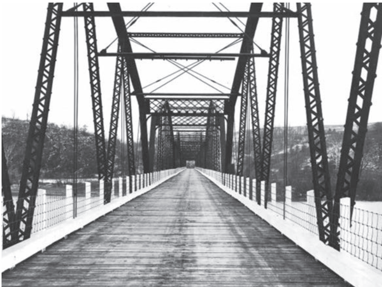
Taken in December 1932, this view of the old iron bridge looks south into Virginia. After a dusting of snow, it depicts the bridge's upgraded wood and wire parapet rail. The truss system was manufactured by the Youngstown Bridge Company of Youngstown, Ohio in 1893.
