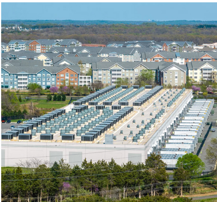
Data centers near residences in northern Virginia.
