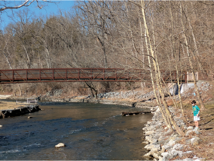
The footbridge over Antietam Creek.
